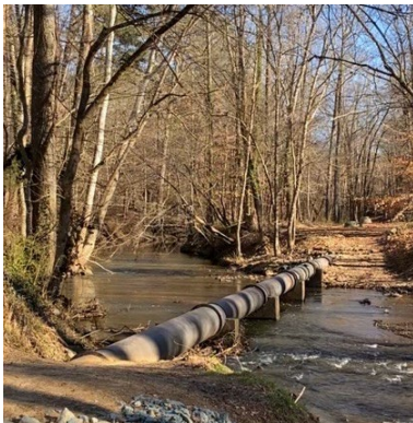
Figure 7 Aerial sewer line crossing Morgan Creek
