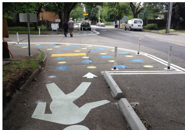
Figure 19 Public art, flexible posts, and pavement markings used to highlight traffic calming (radius reduction) at a roadway intersection with a pedestrian lane.
