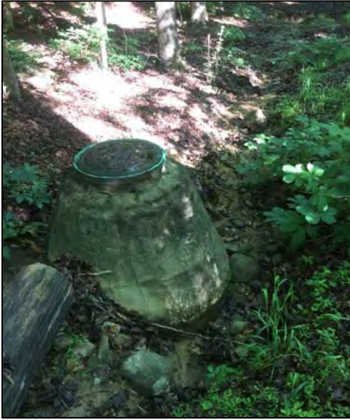
Picture 6-9: Ridgecrest 1 – Existing Sewer Manhole
