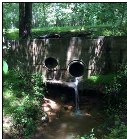
Picture 6-5: Croom – Perched Culvert
